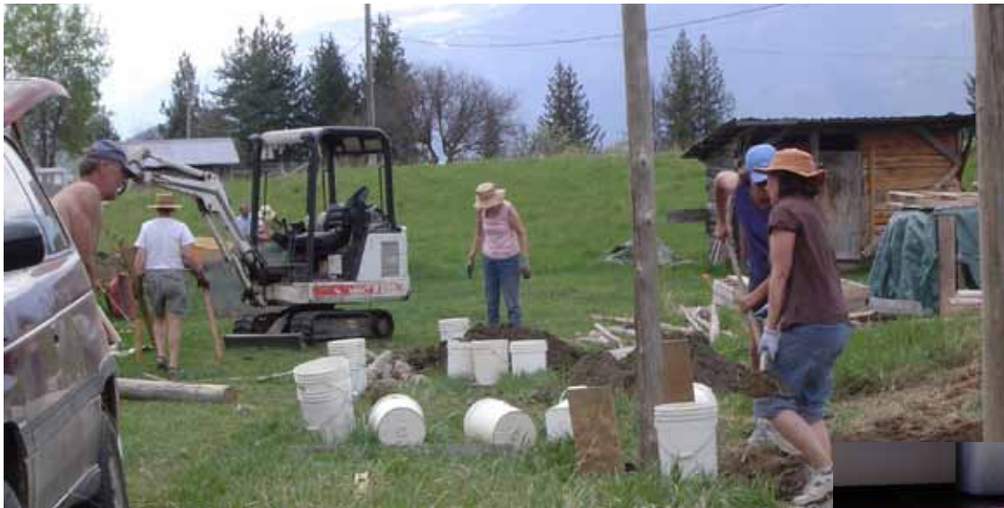
Logs placed in holes after being brought up from the lake to create a fenced area. The buckets are filled with small rocks to put around the poles.
